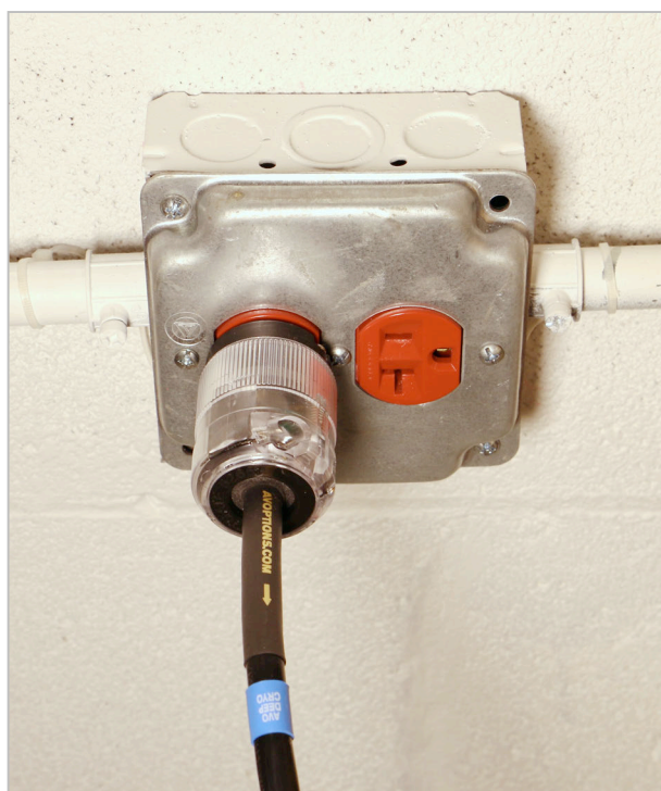
AV Options AC cord in Hubbell Duplex outlet. Outlet mounted in wall box connected to the AC power panel by a dedicated 20A line .
